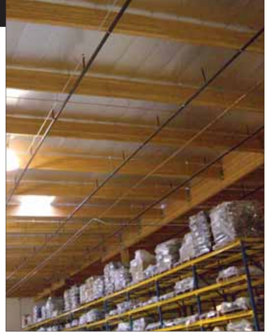
Photo courtesy of The Structures Group.
