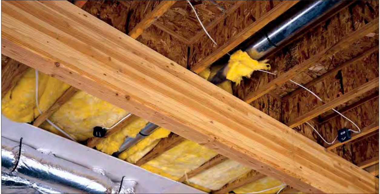
Glulam beam supports second floor I-joist construction.
