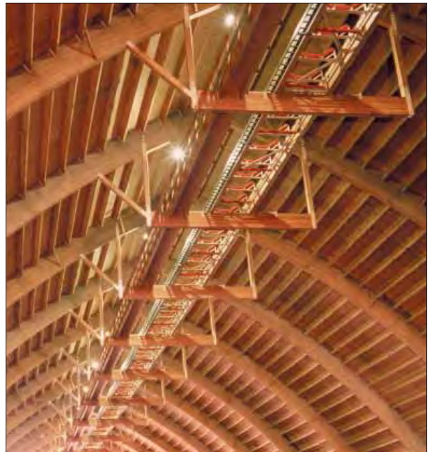
This 236,000-square-foot potash storage building in Portland, Oregon features APA EWS glulam arches.
