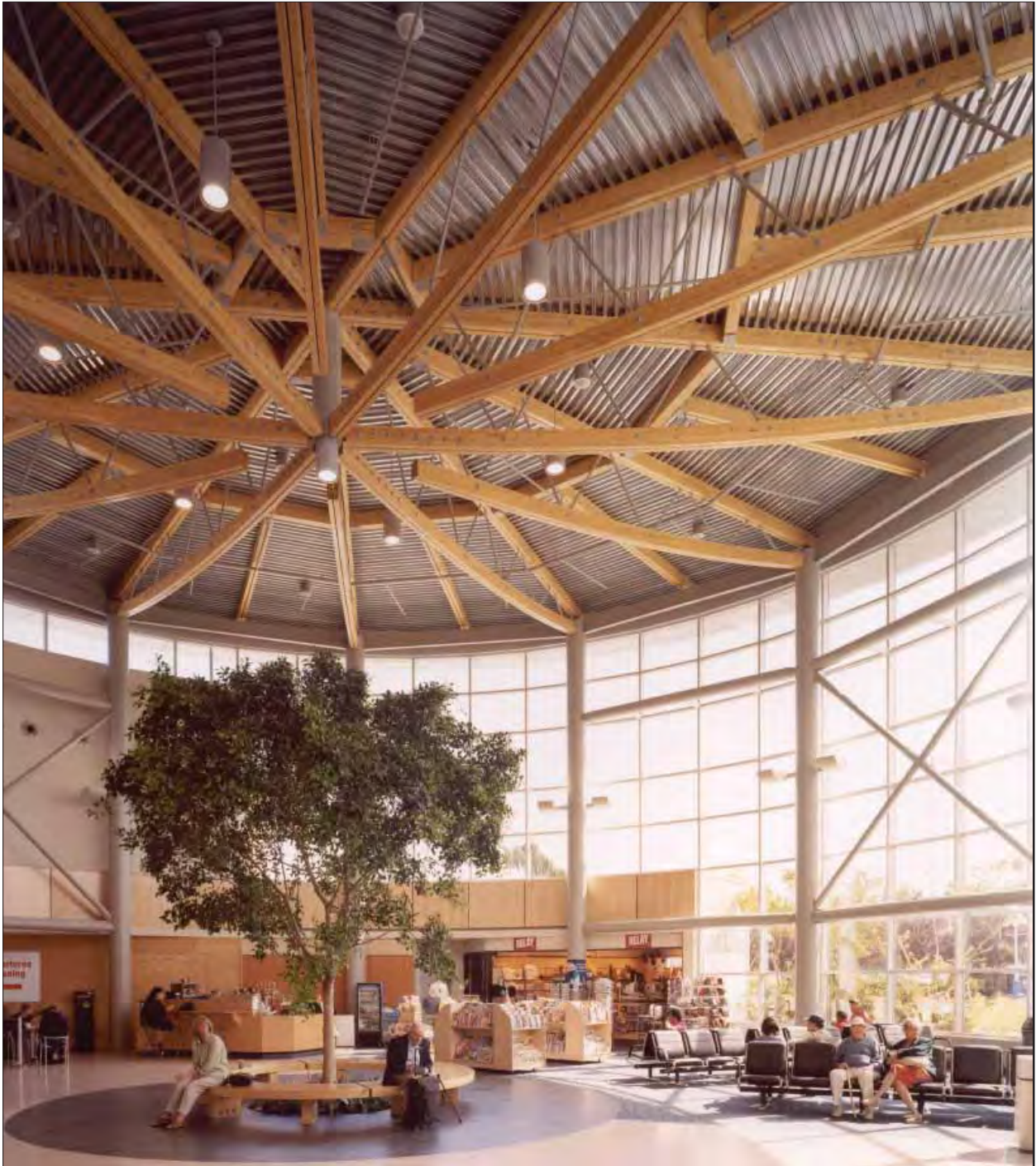
Architects combined spruce glulam with steel and glass to create an innovative and contemporary roof structure for the new rotunda building of the Victoria Air Terminal in Victoria, British Columbia, Canada.
