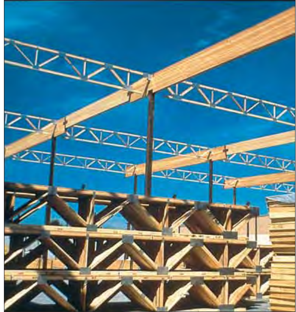
Panelized wood roof with open web glulam trusses and beams.
