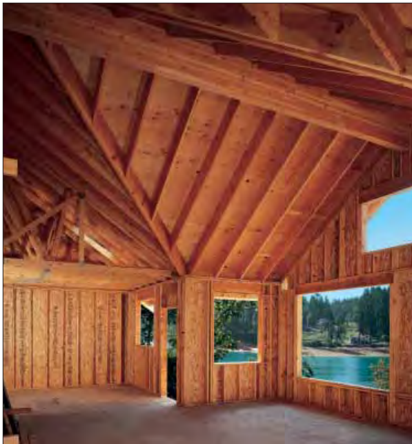
A glulam ridge beam supports the dramatic roof lines in this Western Washington home, shown under construction, left, and finished, right.
