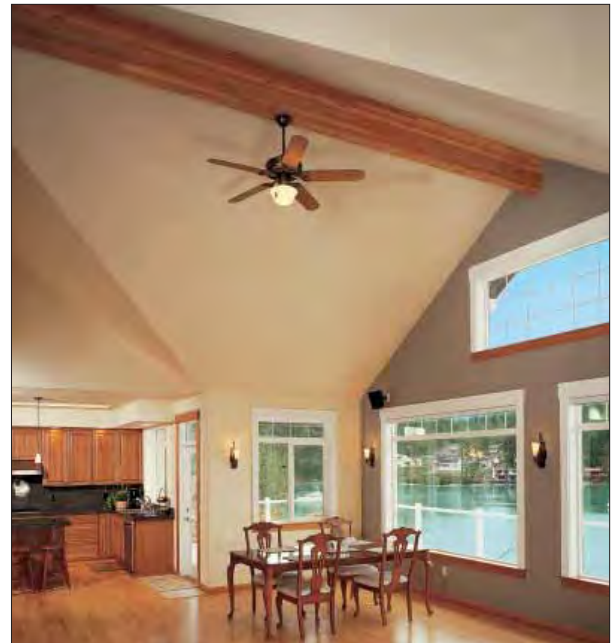
A glulam ridge beam supports the dramatic roof lines in this Western Washington home, shown under construction, left, and finished, right.
