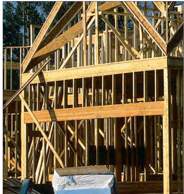
Glulam headers support framing throughout this two-story home.
