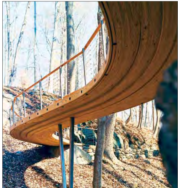
The Madison Footbridge in Madison, Connecticut was prefabricated in six parallel S-shaped lengths of pressure-treated glulam timber.
