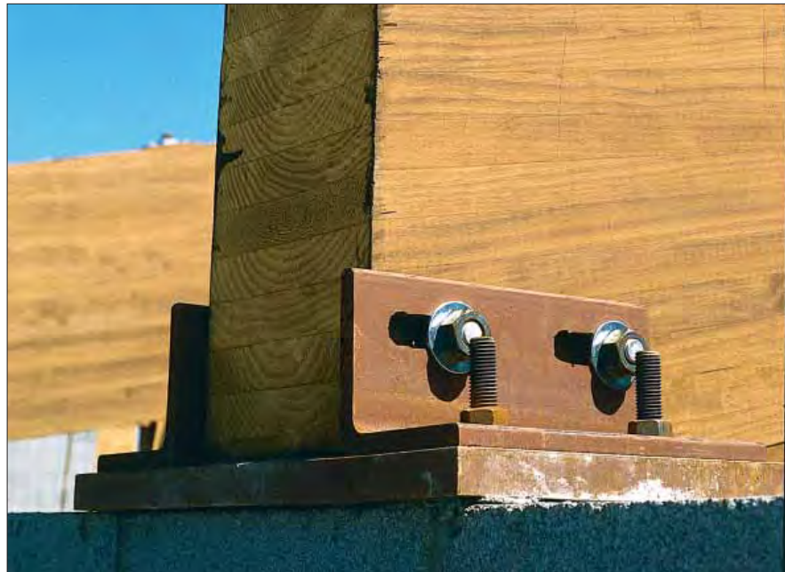
Slotted bolt holes permit horizontal movement of pitched and curved glulam beam.
