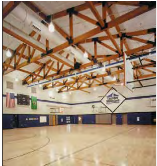
Glulam trusses support the gymnasium roof in Thunder Mountain Middle School in Enumclaw, Washington.
