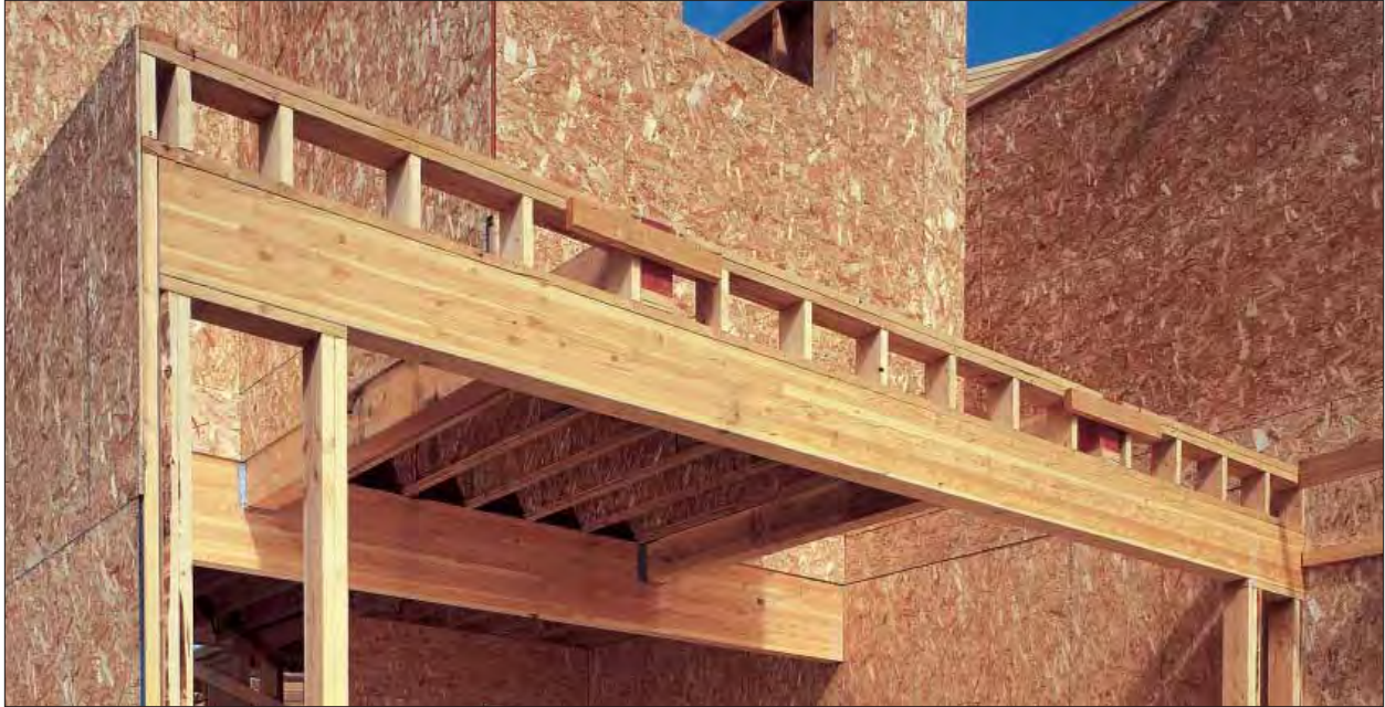
Glulam garage door header extends over adjacent narrow shear wall. (See Figure 4 for further details.)
