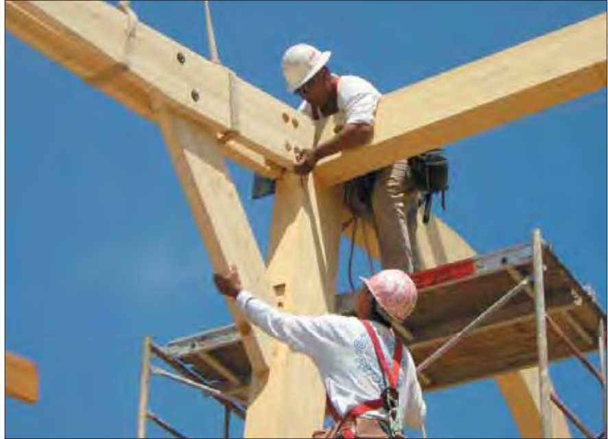
Holes and notches must be precisely located and detailed for architectural appearance and accounted for in the design of beam connections and column capacity.
