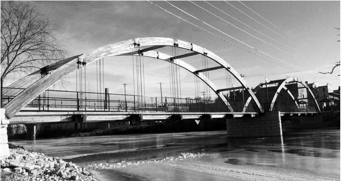
The Milwaukee Street Bridge in Jefferson, Wisconsin features 3-hinged buttressed arches each with an 85-foot radius.
