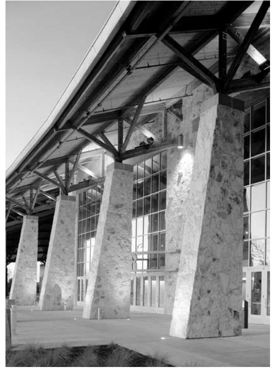
Austin, Texas' Palmer Events Center features glulam trusses attached to a matrix of concrete columns.
